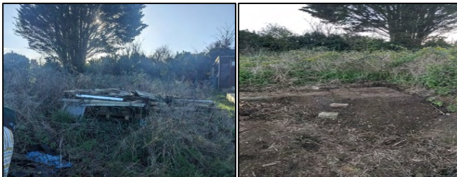
Before and after rubbish clearance
