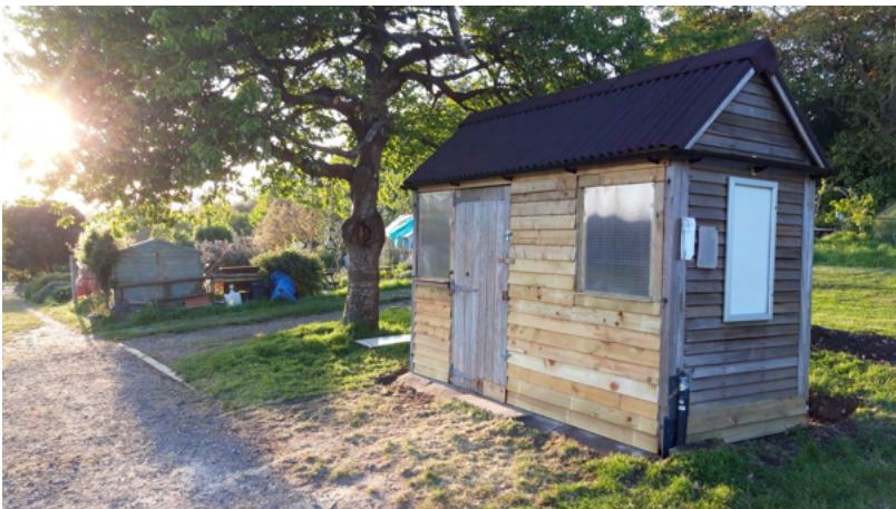
The LCE shed renovated with BAA funds
